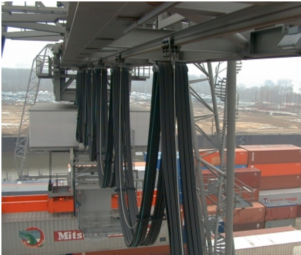
Figure 4-11 Use of the PROFIBUS Cable for Festoons
